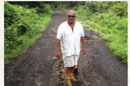
Tommy Capossela assessing the damage on Old Sleepy Hollow trail
