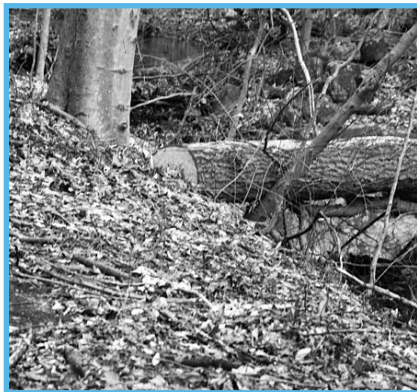
Debris along the trail blocking culverts
