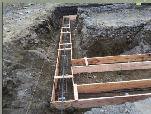
Construction crew laying the concrete forms for the shop’s foundation.
